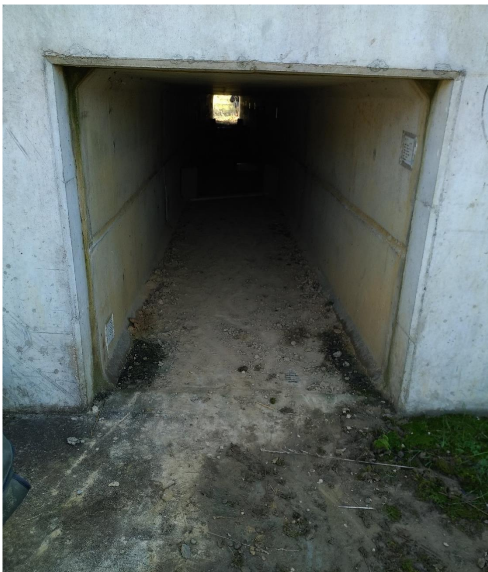
Figure 1: Tunnel implemented under a railway as mitigation for the amphibian community (square concrete culvert 21m length, 1 m high, 1 m width)
